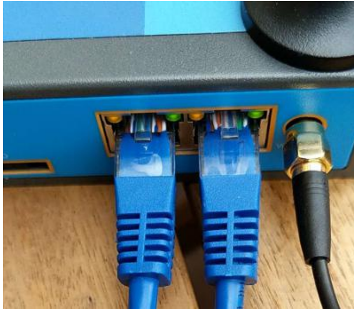
Figure 2.4 Connect Ethernet cables
