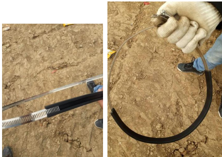
Figure 58 Wrap the anchor ear with rubber strip
