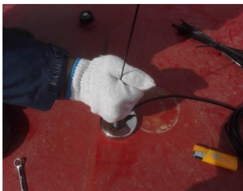
Figure 32 Slightly pull the antenna to check if it is securely adhered
