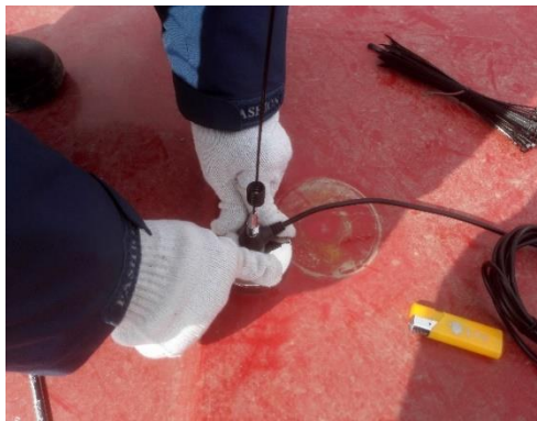
Figure 30 Remove the protective film of the double faced adhesive tape on the antenna pedestal
